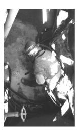
Note the clean, low dust environment enjoyed by this pliant media blaster on a checkered platform deck plate. dust in two ways. First, it flattens on impact, acting like a blanket, which inhibits the ricochet of the airborne paint and contaminants. Second, it traps paint and contaminants in its porous structure. The result is a significant reduction of airborne dust.
