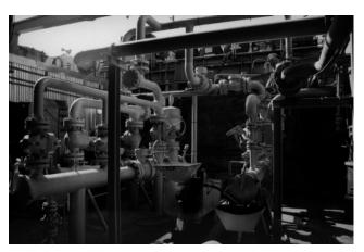
Blasting near a "Pig Launcher" on this platform required little equipment wrapping and containment due to pliant media technology's low rebound and low dust attributes.
